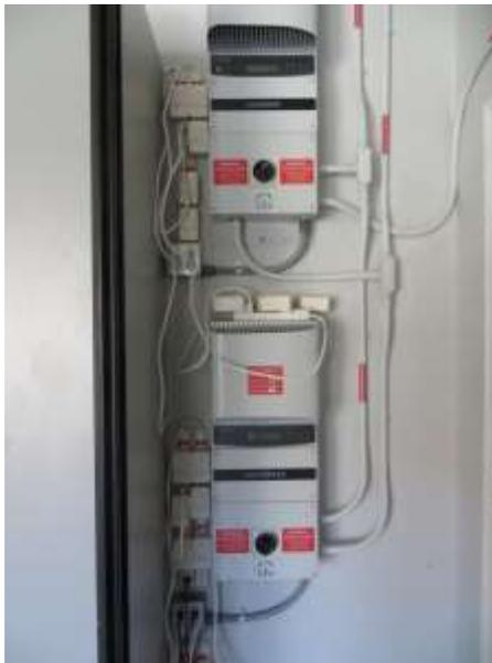
Figure 3 Solar Inverters with filters.
